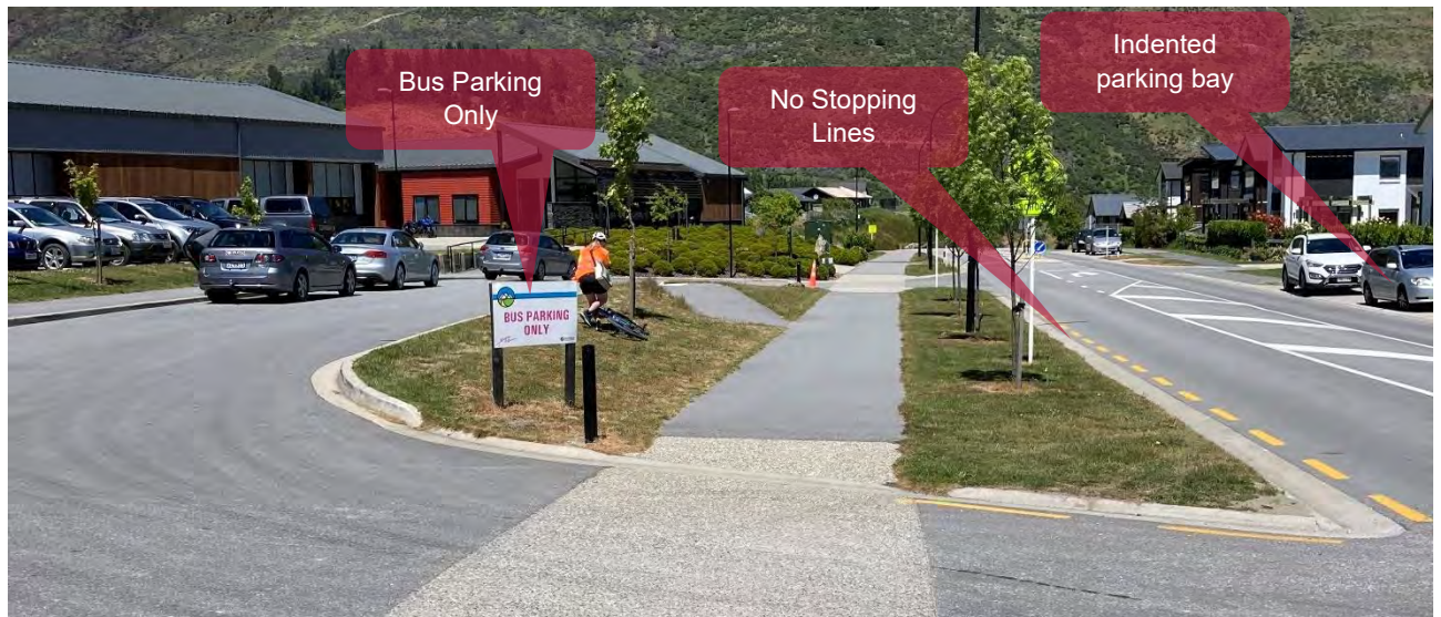
Figure 4.18 Stalker Road School Frontage
