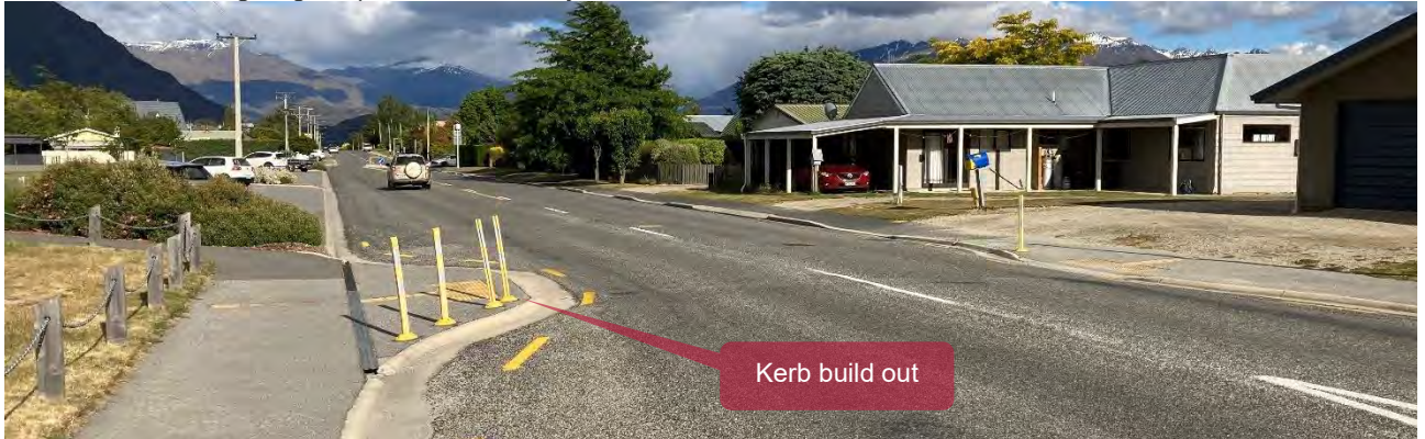
Figure 4.24 Kerb build out with tactiles
