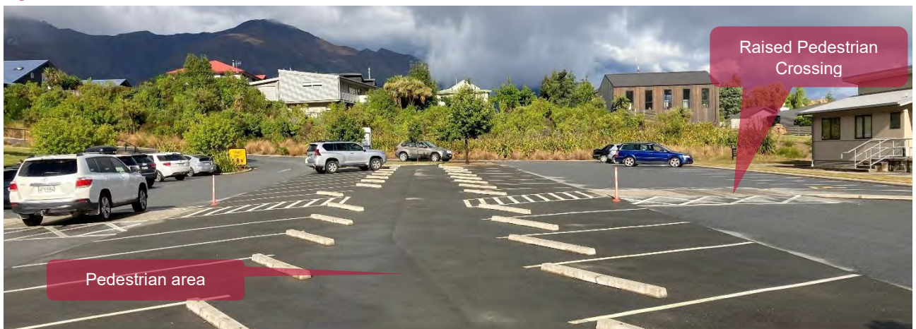
Figure 4.35 Totara Terrace Car Park
