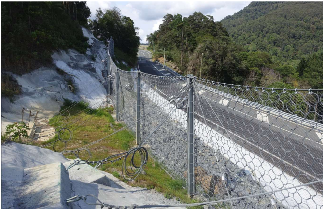
Figure 4.1: Schematic representation of a typical debris flow barrier. (Source GeoBrugg)
