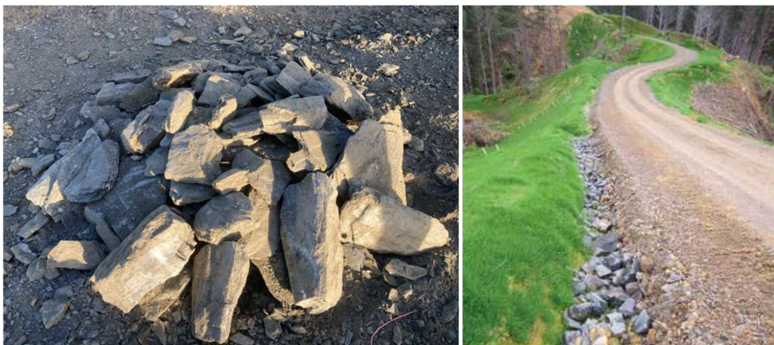
Photograph 4.1: Site-won material available to be used as drainage ditch riprap (left). Right: a recommended example riprap configuration from the NZFREM
