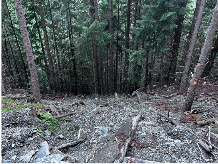
Photograph 6. Upper Debris Field Looking Downhill Towards the First Bluff. Source – Sean Dent 25.01.24.
