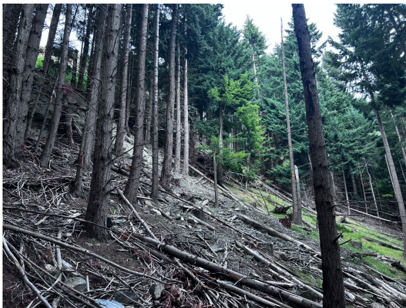
Photograph 4. Upper Debris Field. SEL Lease Area in the Top Left Corner. Source – Sean Dent 25.01.24.
