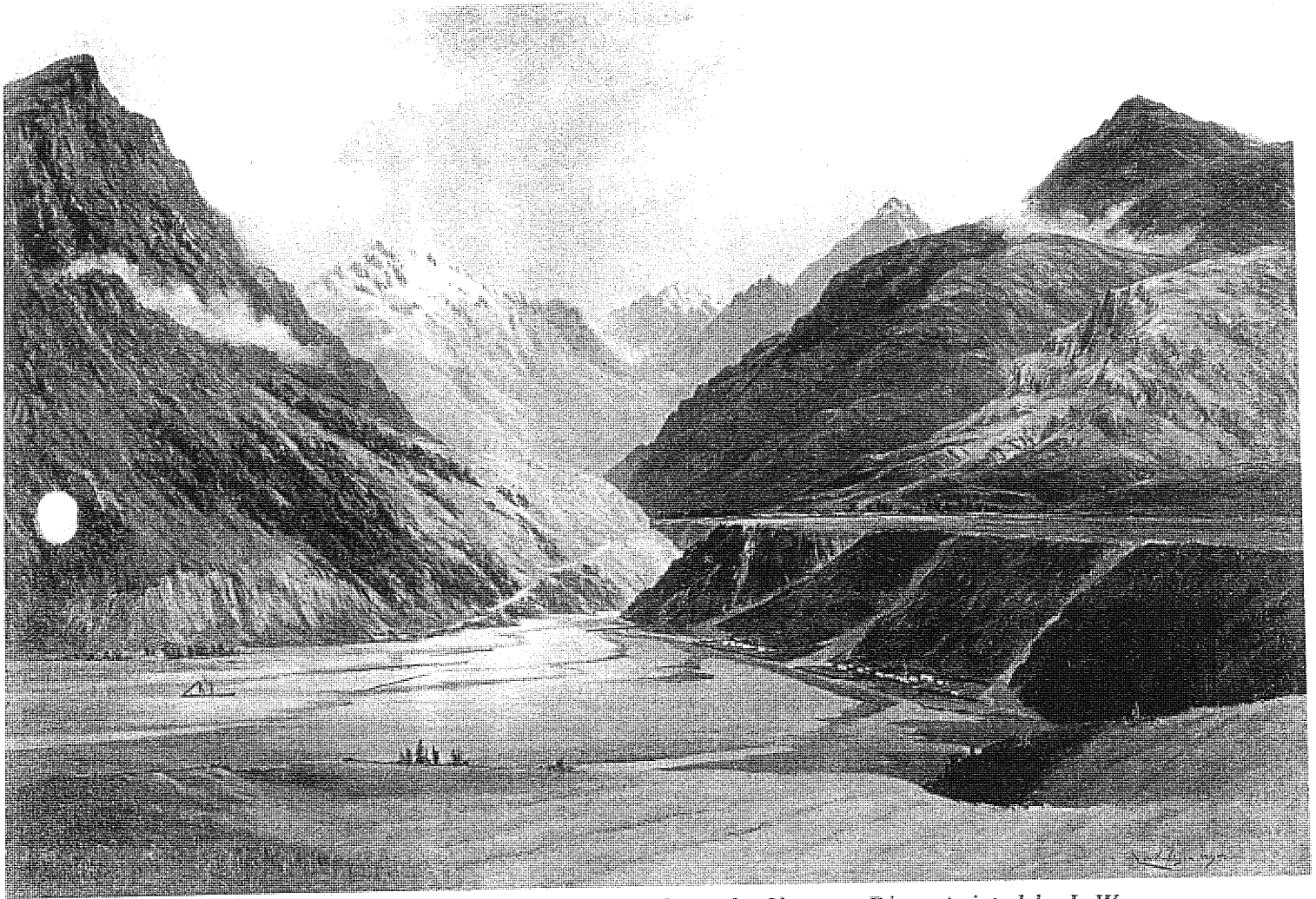
CHOIE SEW HOY'S dredging claim at Big Beach on the Shotover River, painted by L. W. Wilson in 1895. The view is upstream, and beyond the gorge in the middle of the picture are Arthurs Point and Morning Star Beach. Downstream, out of the picture to the left, are Tucker and Talisman beaches. All these beaches were dredged by the Sew Hoy Big Beach Gold Mining Co., but the richest and most extensive deposits were at Big Beach itself. [Dunedin Public Art Gallery]
