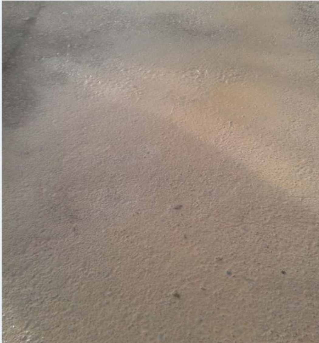
Figure 3 Aggregate wetted down during compaction to achieve 98% of MDD – note no compaction depression lines
