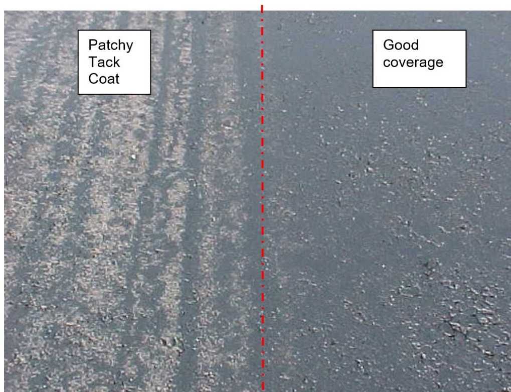
Figure 4 Tack Coat Application Examples
