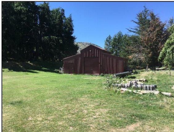
Plate 5: Newly built storage shed
