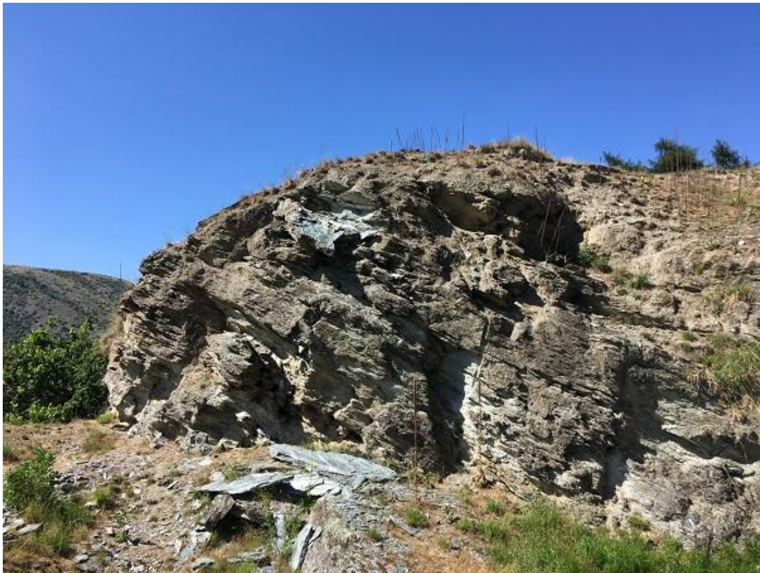
Photograph 3. Local small scale recent rock fall from a schist bluff.
