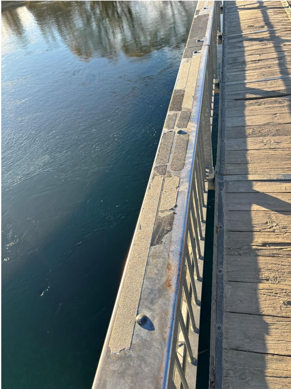
Figure 8 Grip Tape Installed on Preferred Jumping Zone
