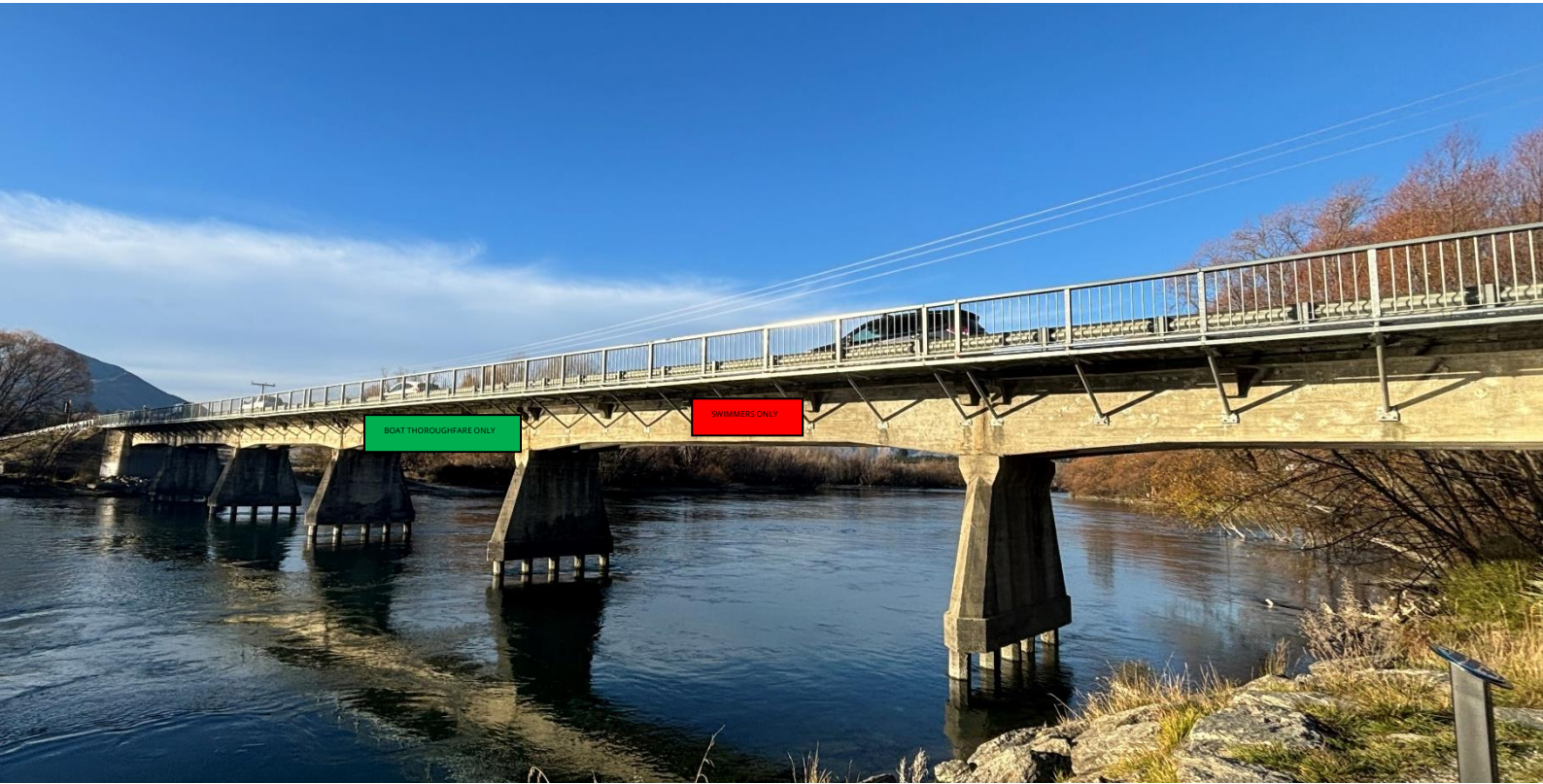
Figure 9 Exemplary Bridge Signage Concept – Green Sign (Boat Thoroughfare Only), Red Sign (Swimmers Only)
