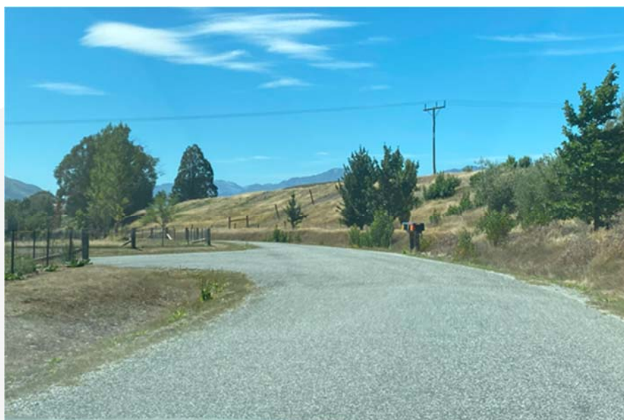
Photograph 6: 'Tee Intersection' With Main Roadway Curving Left
