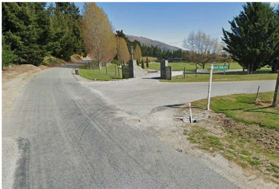
Photograph 1: Morris Road / Black Peak Road Intersection
