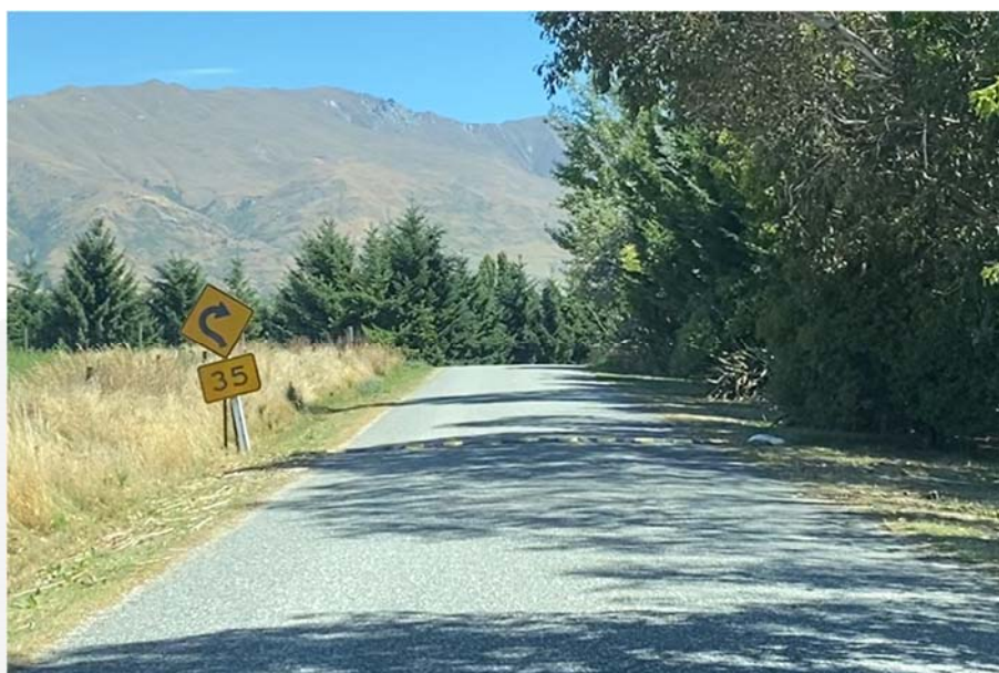
Photograph 4: Curve Warning Signage for Westbound Drivers and Hump
