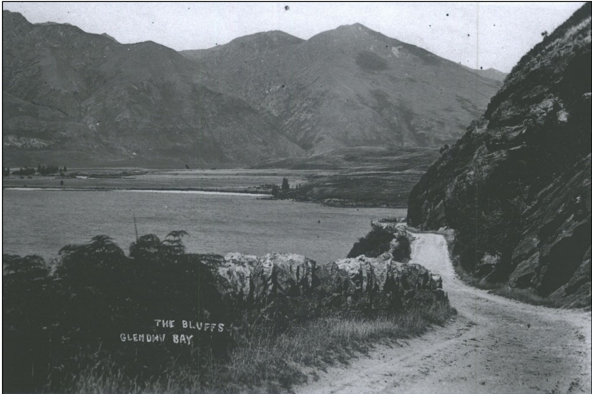
Figure 19. The Bluffs at Glendhu Bay, undated. 176
