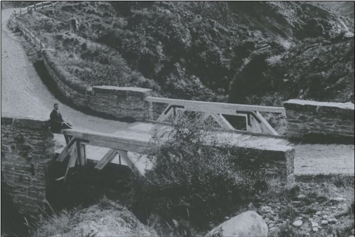
Figure 13. McChesney's Bridge circa 1903. 113
