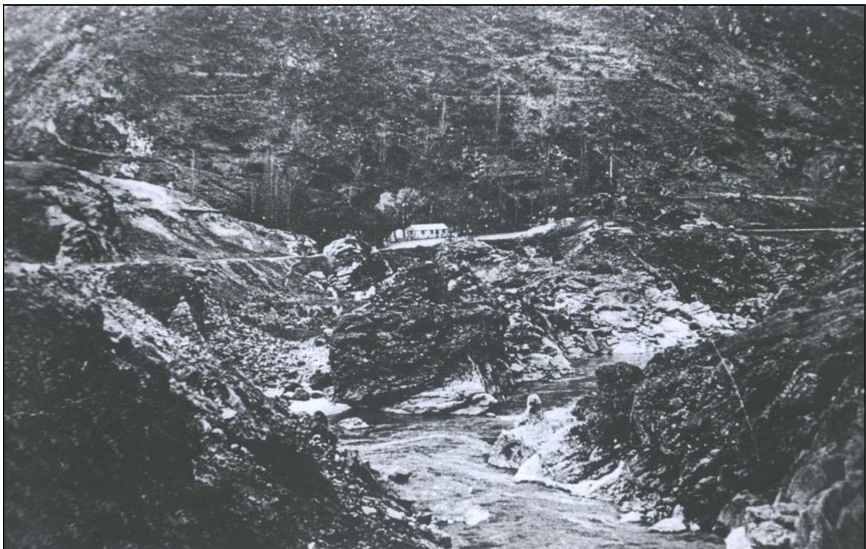
Figure 7. Kirtleburn Hotel and shop pre-1880s, situated adjacent to the Roaring Meg. 75
