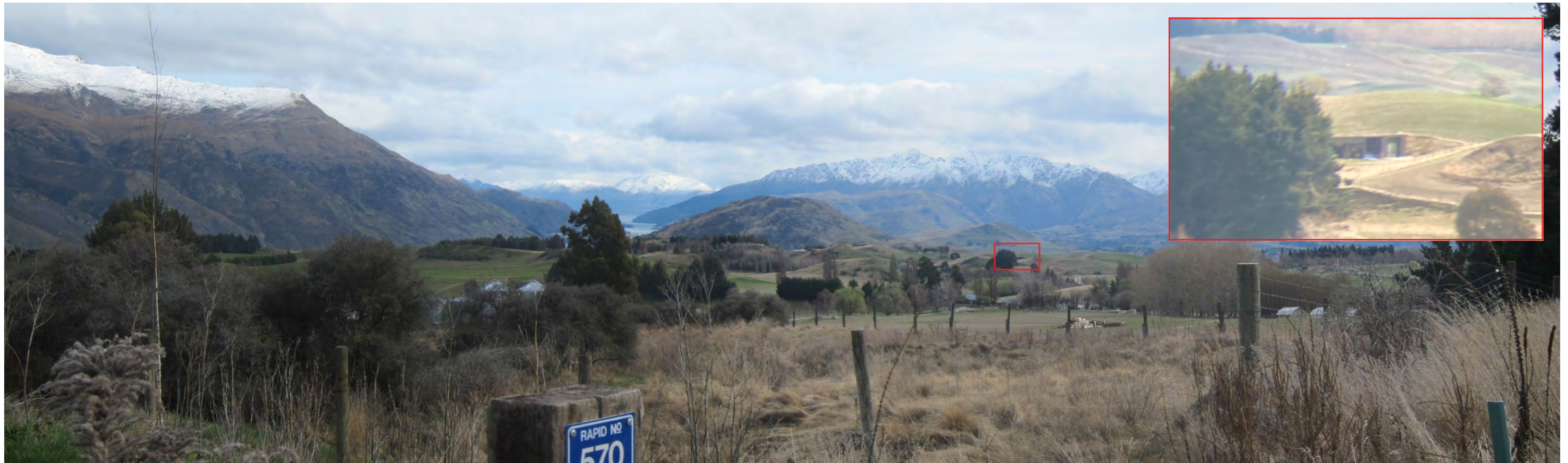
Viewpoint 3: Looking towards the site from Crown Range Road. The established shed can be seen from a distance of over 2km.
