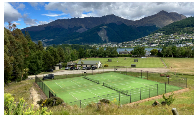
Figure 10 - View looking towards Queenstown with the park's tennis courts, informal parking area and the croquet club in the foreground
